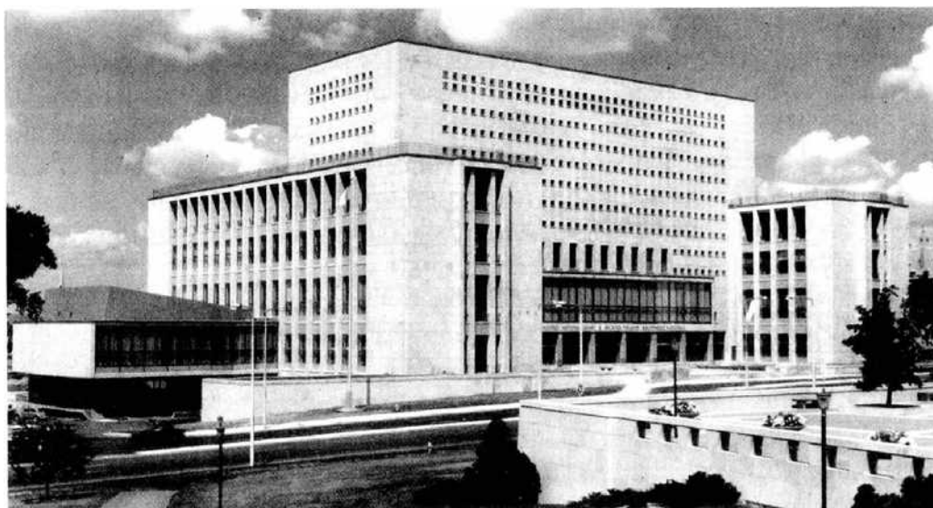
FIGURE 1. National Library and Archives Building, Ottawa, Canada.
