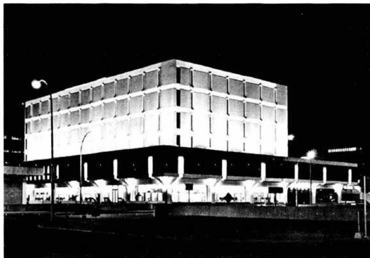
FIGURE 5. Main building of the Edmonton Public Library. (Courtesy Morton Coburn. Photograph by Charles H. Machtans.)
