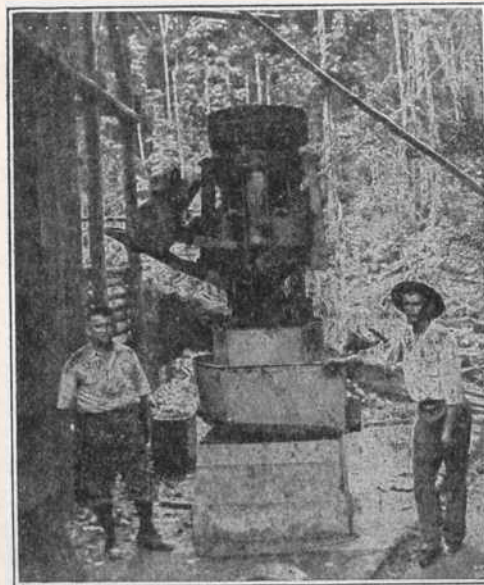
FIG. 119.—Latest model of a Straub 10-stamp mill with capacity of 12 to 15 tons ore per day.
