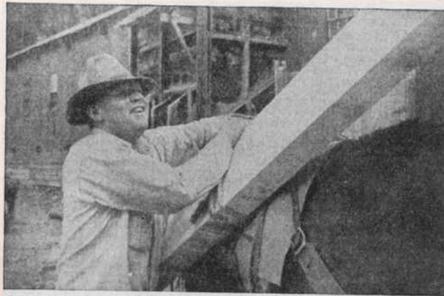
FIG. 7.—Tying on a 3- by 12-inch board. Boards and small pieces may be nailed together. (Courtesy of George O. Argall, Jr.)
