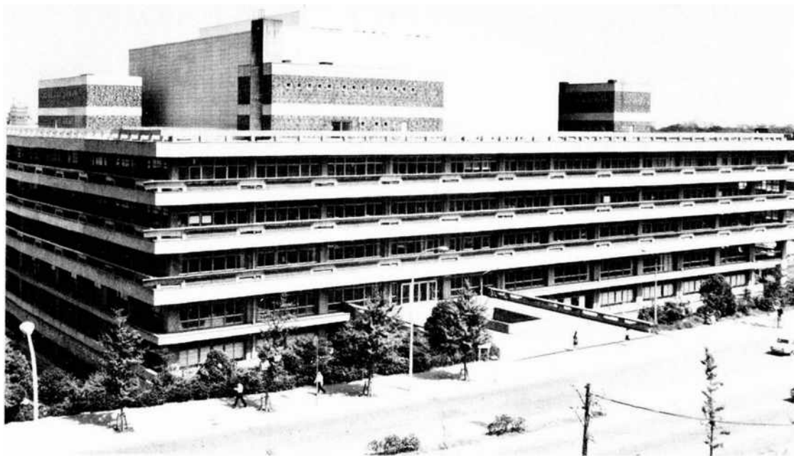
FIGURE 1. The National Diet Library. Because the building is built on a slope, the bridge at the front leads to the third floor. The upper, white part is the stack area.
