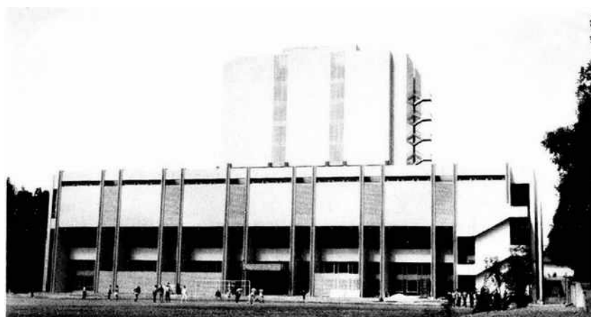
FIGURE 2. The Central Library and Documentation Centre, University of Tehran.
