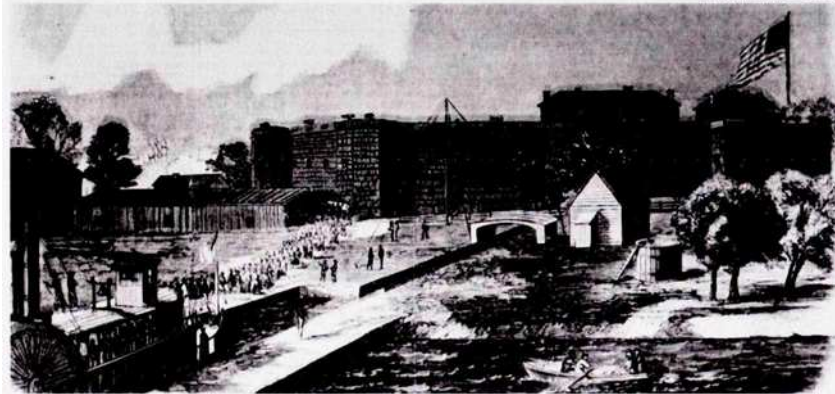
Fort Delaware became a prison for captured Confederate soldiers during the Civil War (1861-1865). The pentagon-shaped fort is located on Pea Patch Island in the middle of the Delaware River. The fort was originally built for coastal defense in 1859.
